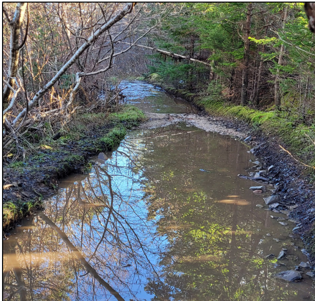
Photo 4-2 – Abandoned CN Railway Ponding
