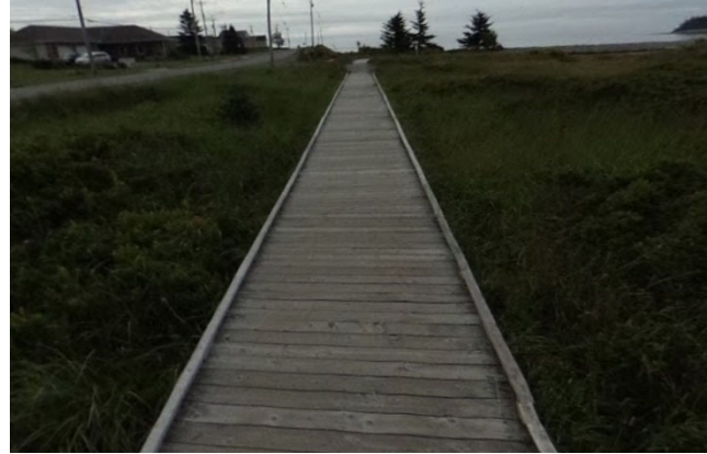
Photo 3-4: Shore Road Boardwalk Facility
