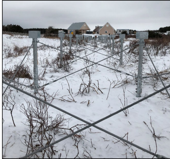
Photo 3-2: Helical Piles for Boardwalk
