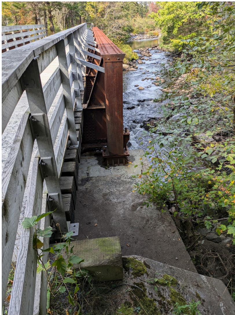
Figure 1: Example of two posts that require bracing
