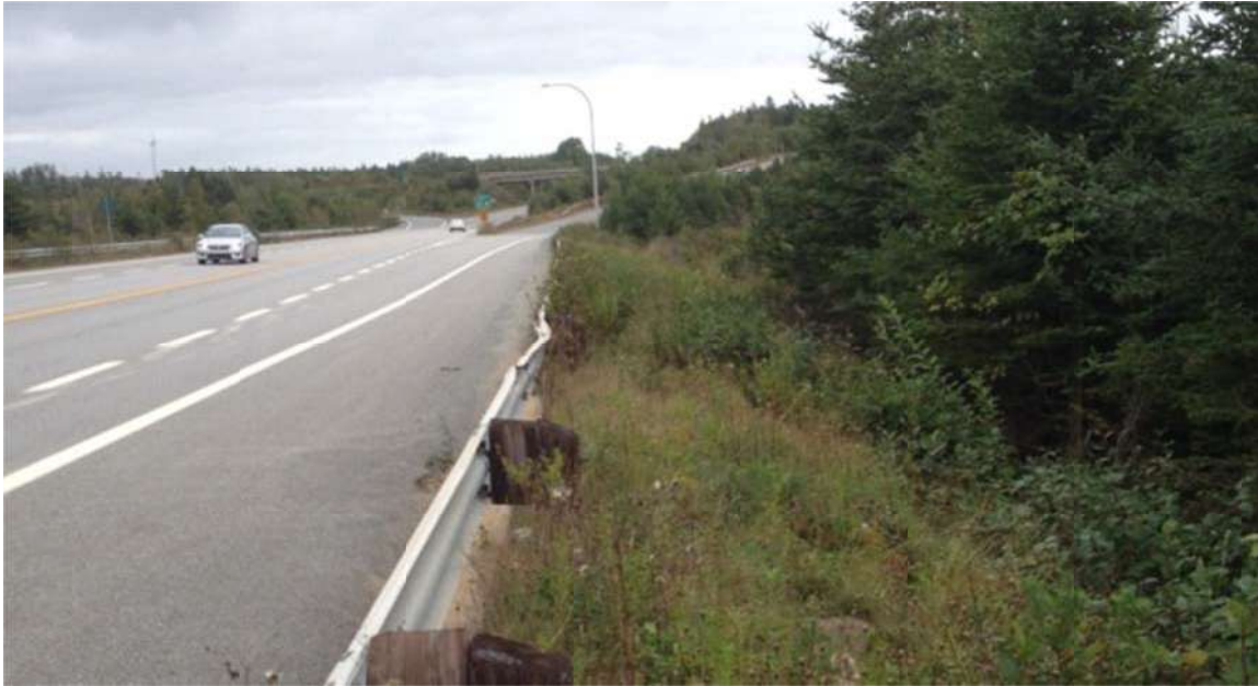
Photo 5-14: Looking east toward the Exit 21 Off-Ramp
