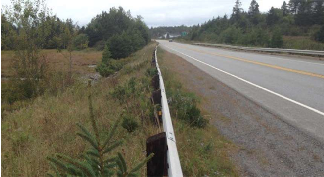
Photo 5-3: Looking west on Highway 107
