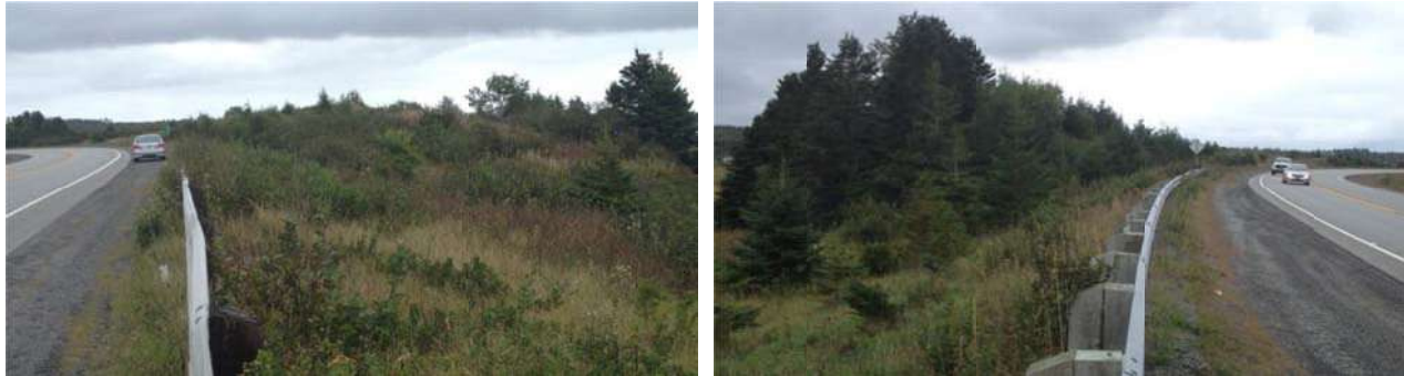
Photo 5-6 and Photo 5-7: Looking east (left) and west (right) on Highway 107
