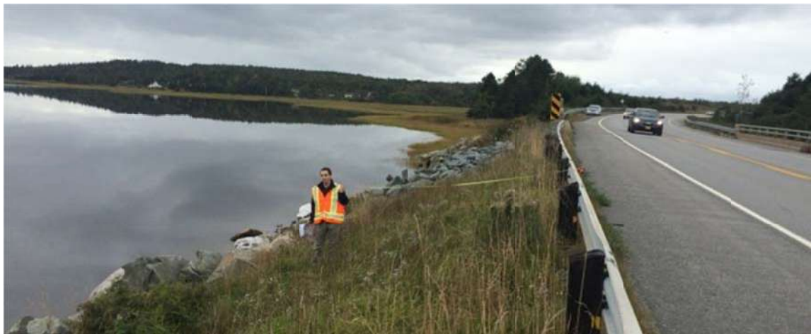
Photo 5-9 Looking west on Highway 107
