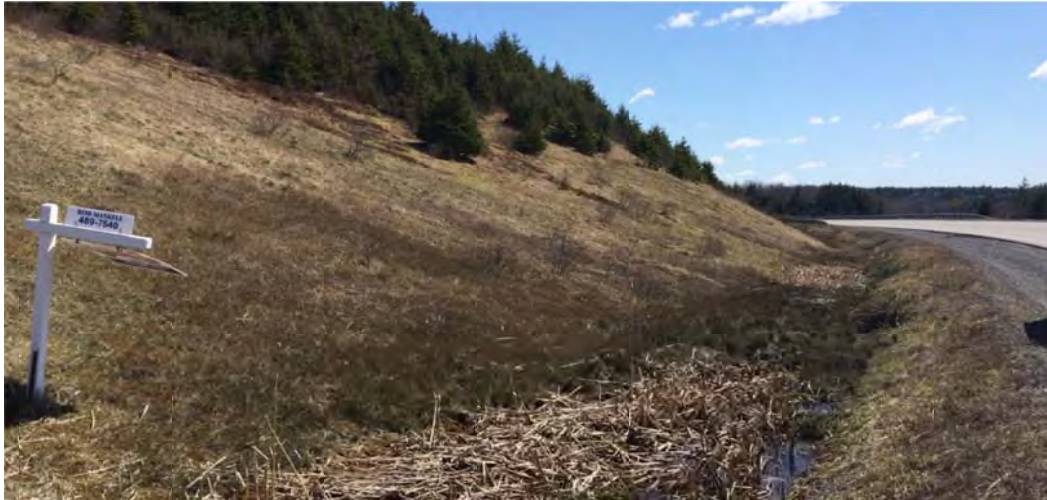
North side of Highway 107
