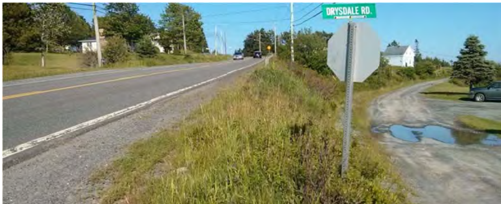
Trunk 7 at Drysdale Road
