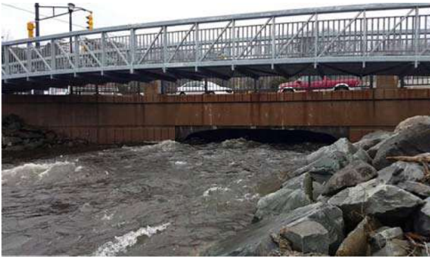
Active transportation Bridge in Bedford, NS.
