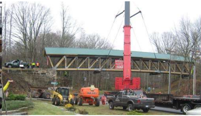
Example of a Pre-fabricated bridge structure being hoisted in place.
